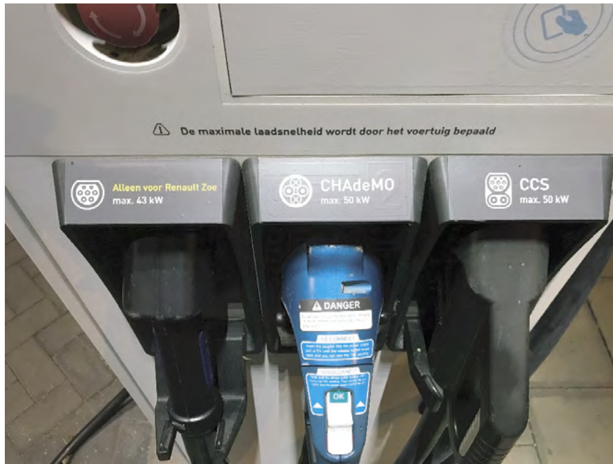
Figure 15. A fast charging installation with multiple technology options
