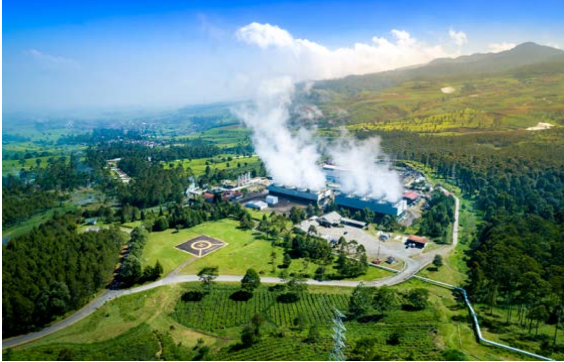
Wayang Windu Geothermal Power Plant, Bandung, Indonesia. Photograph: Shutterstock
