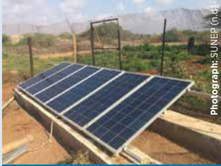
Solar panels connected to water pump for deep wells, replacing old diesel water pump
